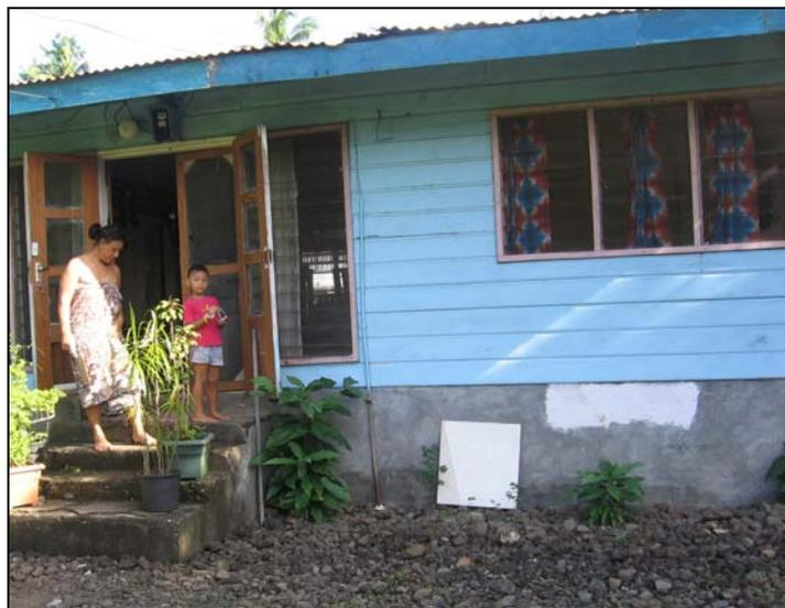
*Figure 22. A raised threshold prevents damage from minor flooding.*
