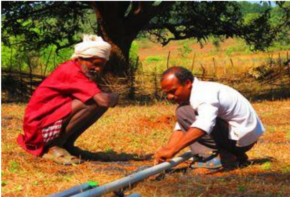
Installation of the Driptech system
