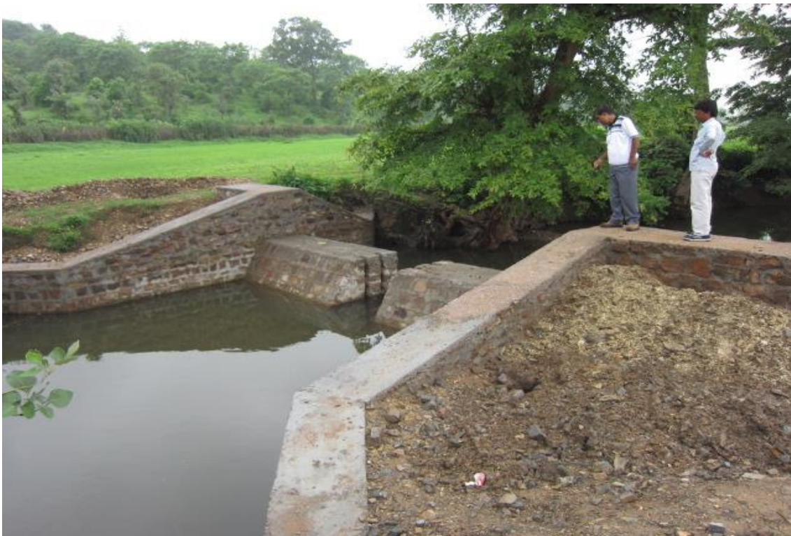
A dam constructed by Haritika near Chandanpura
