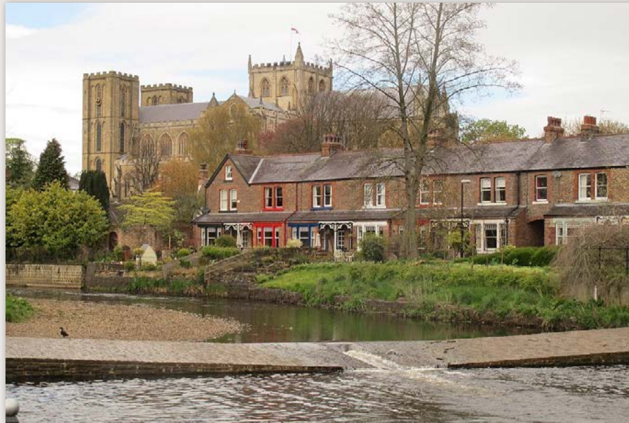
Figure 10: Alma Weir, Ripon. The weir was rebuilt in 2010.
