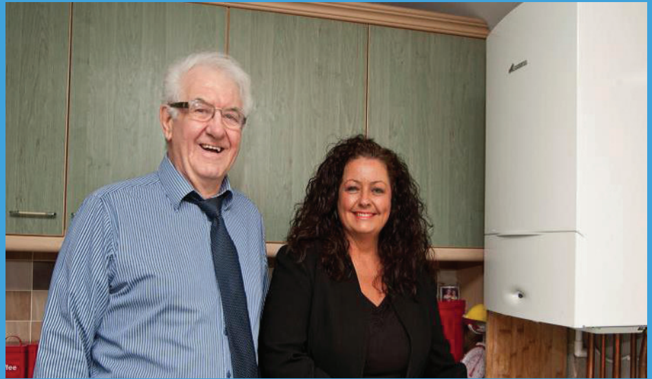
Warm Zones' Michelle Rodgers with client Mr Baldwin, who had a new boiler installed free of charge
